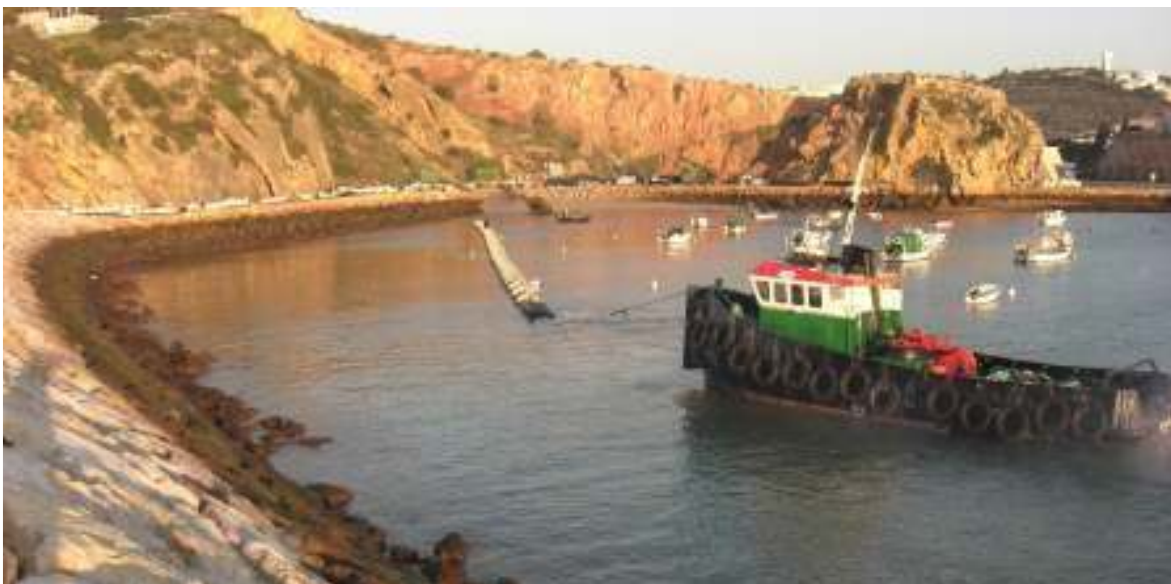
Reboque de conduta (Albufeira, 2009)
